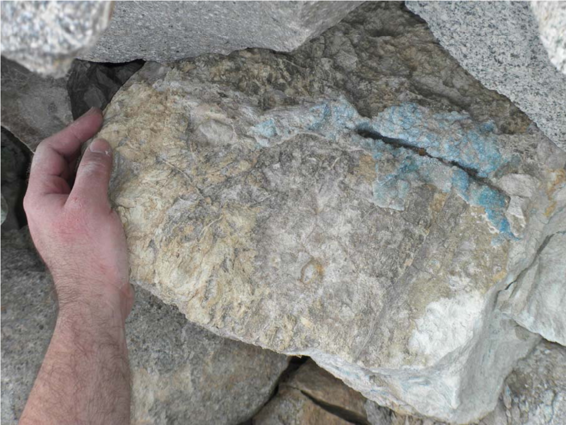
The “mousetrap rock” had a huge vein of blue kinkite running through the middle. It was also underpinning a series of huge boulders up the hill. We engineered alternate support for the uphill boulders and set to cracking.
